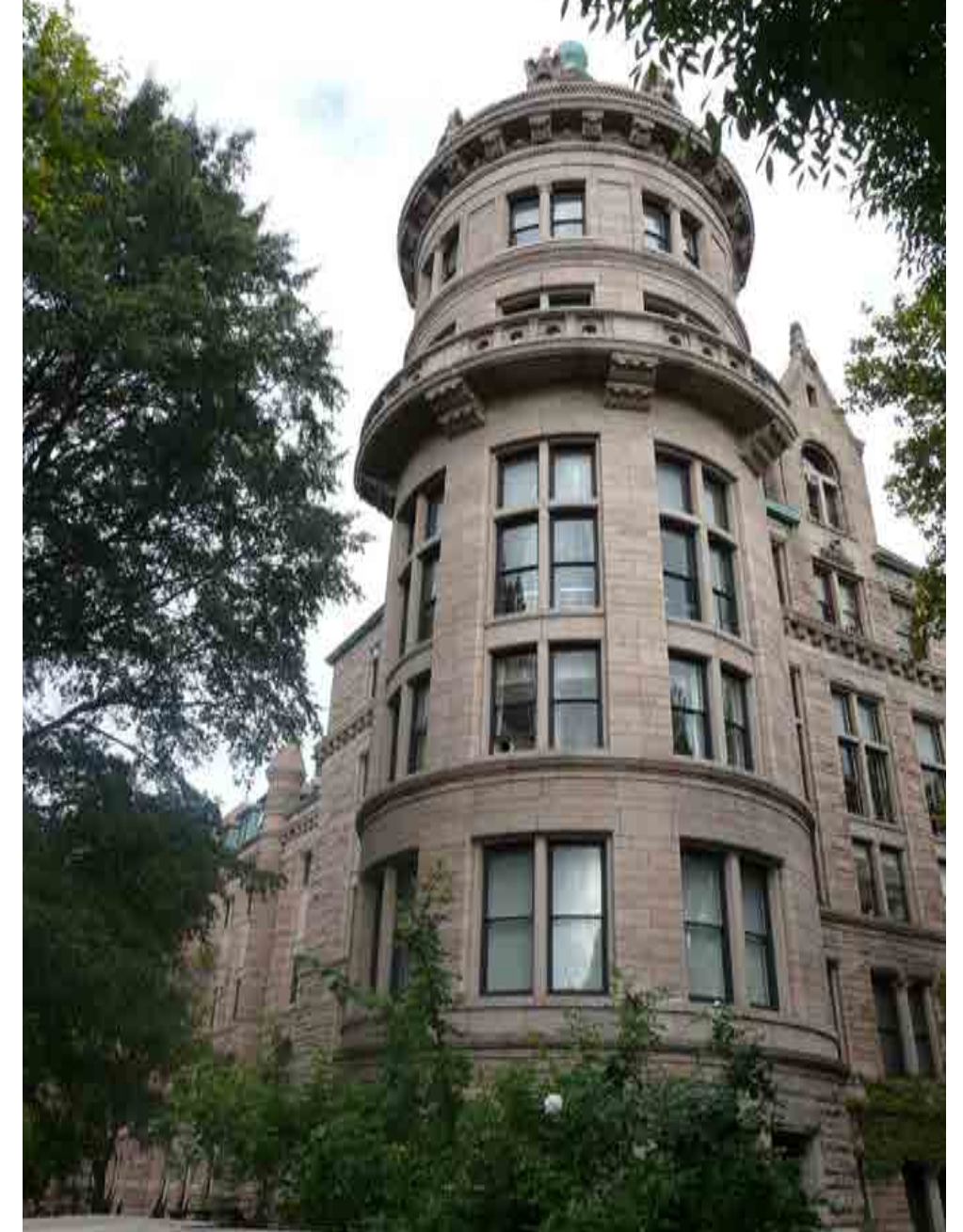
View of Building 6
