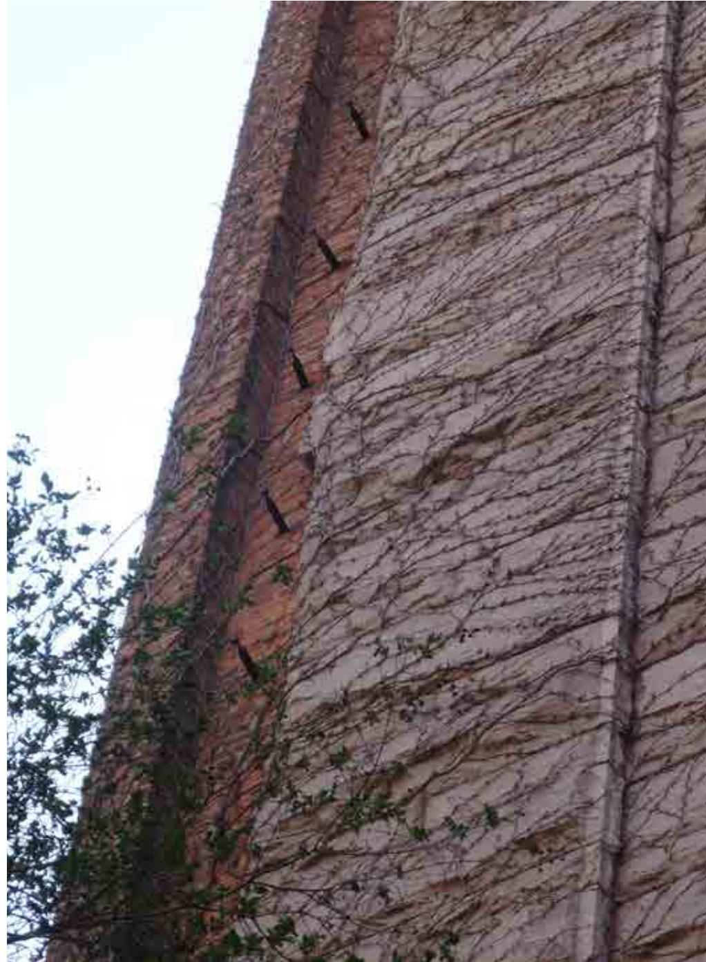
View of Building 8 corner detail
