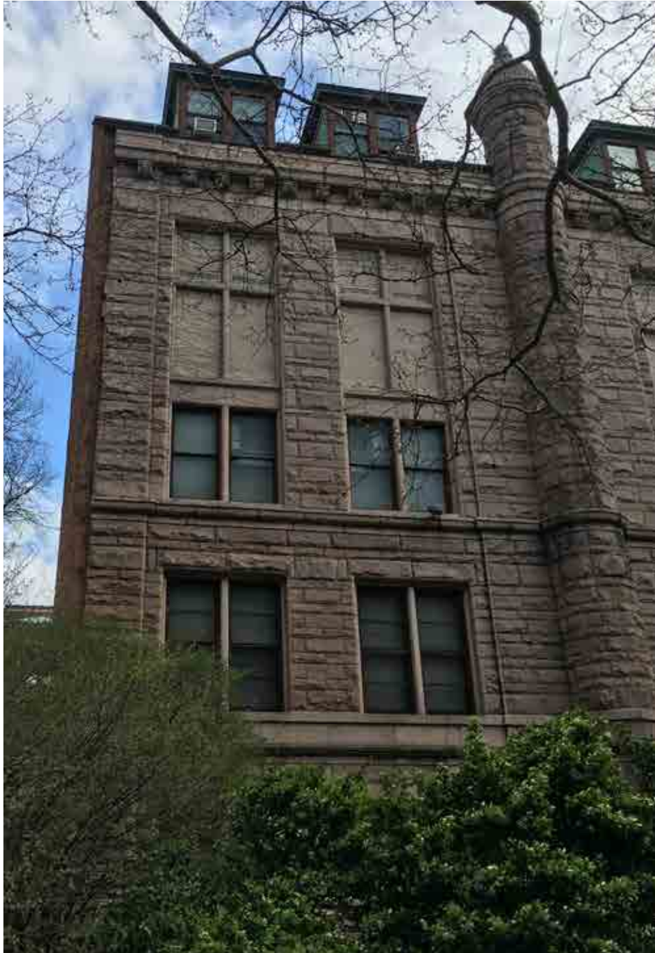
View of Building 8 West facade
