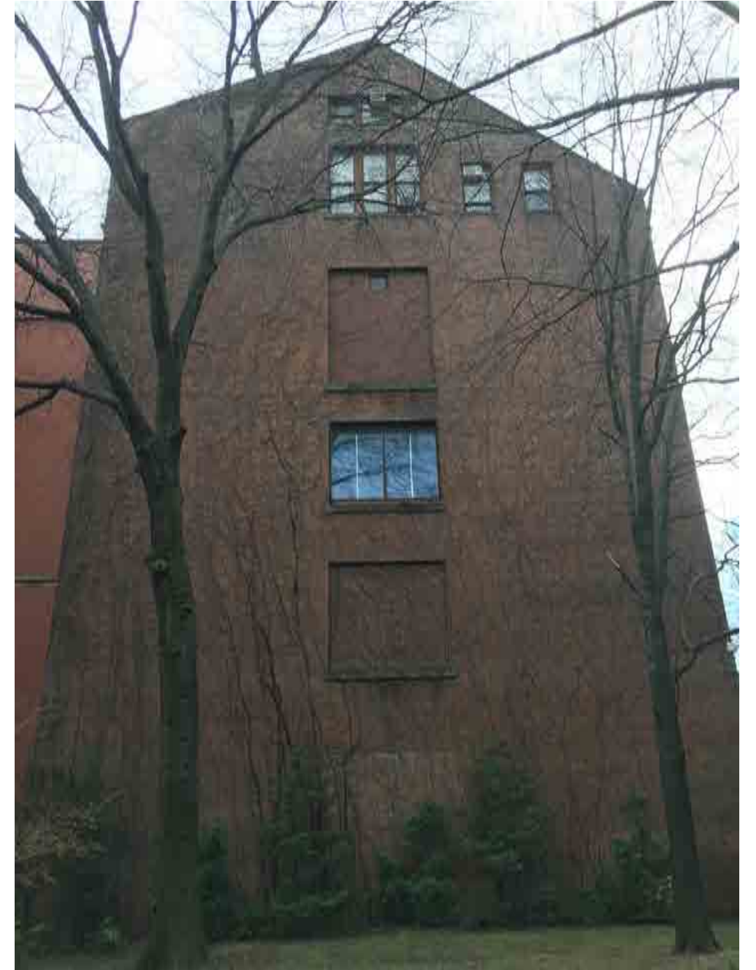
View of Building 8 North facade
