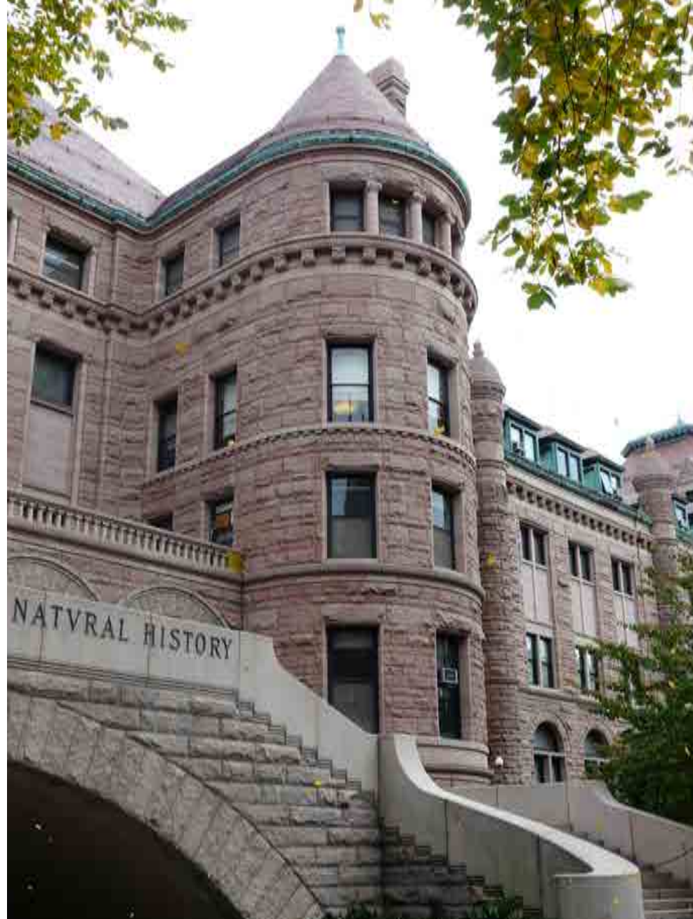
View of Building 2
